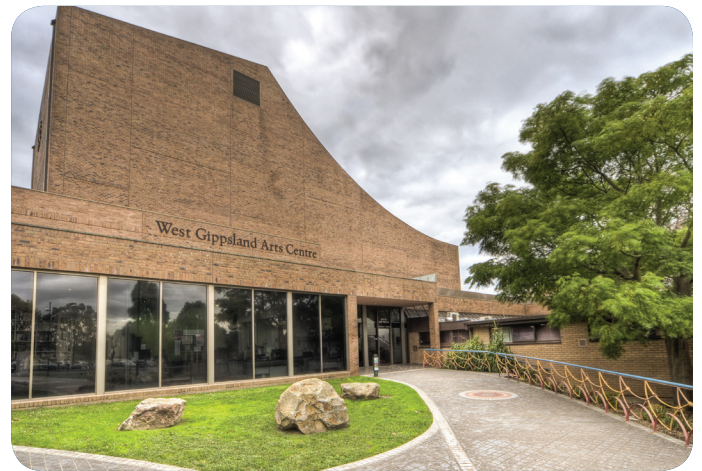
The current entrance of the West Gippsland Arts Centre.
